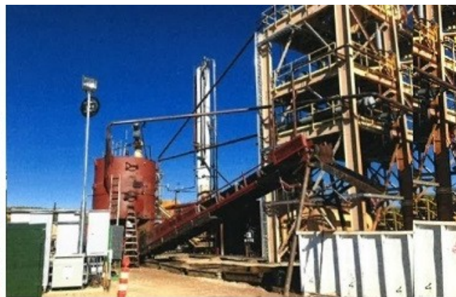
Product Storage Tanks
